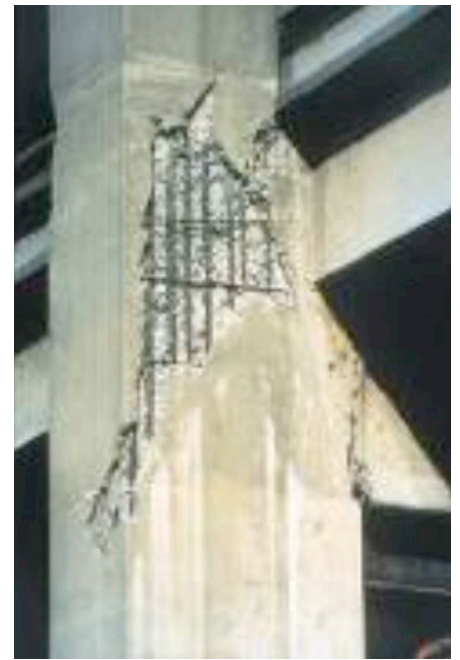
Lap splices transfer their load through the concrete and will fail as concrete cover degrades.
